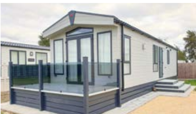
Toughened Glass in Grey Glass Clamps
